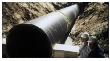
Three lengths of Weholite were extrusion fused, on site, to form one continuous 122 ft. long section. The fused section was then lowered into the deep trench using two excavators equipped with nylon slings. DPW Director Anthony Hayes commented, "We're convinced Weholite is great pipe for this kind of application, and should last for many generations." Tim and Mike White, of White Brothers, commented that the job was challenging and it was fun too!
